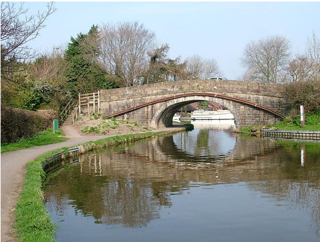
Moss Lane Bridge looking north ( www.canalwalking.co.uk )
