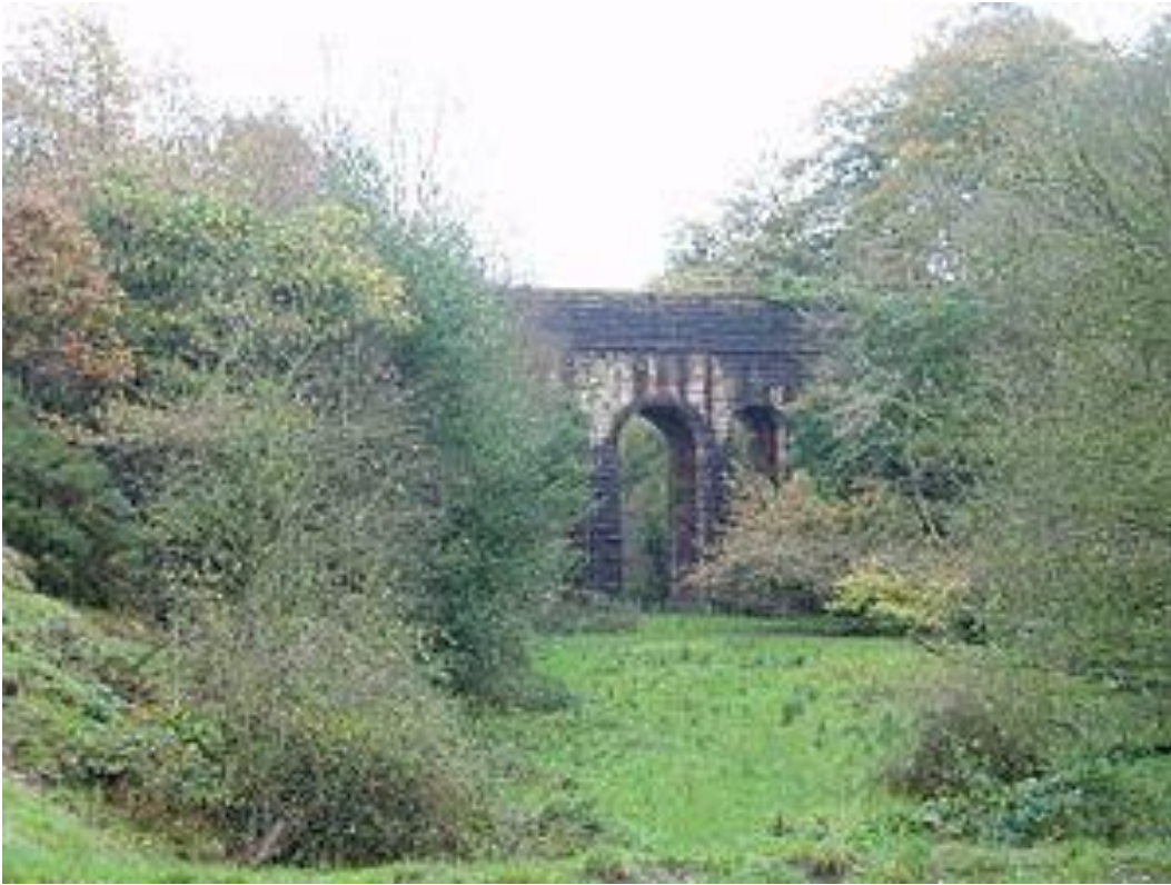
Thirlmere Aqueduct viewed from canal bridge 87, near Higher Wheelton (By Charles Rawding, CC BY-SA 2.0)
