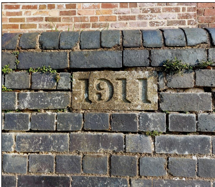
The date stone at Diglis Lock which may refer to an engine house reconstruction
