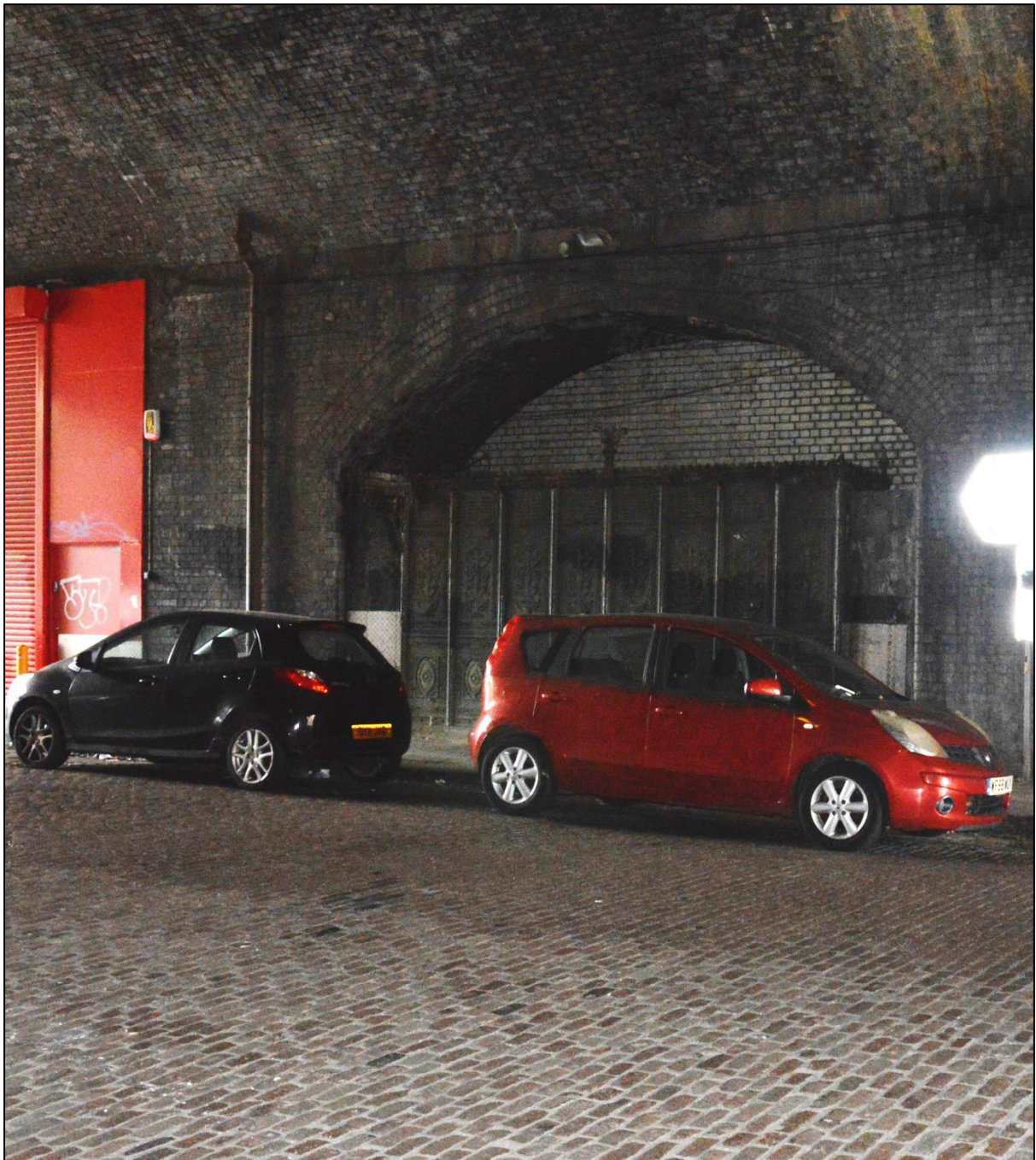
The iron urinal and stone setts in the road
