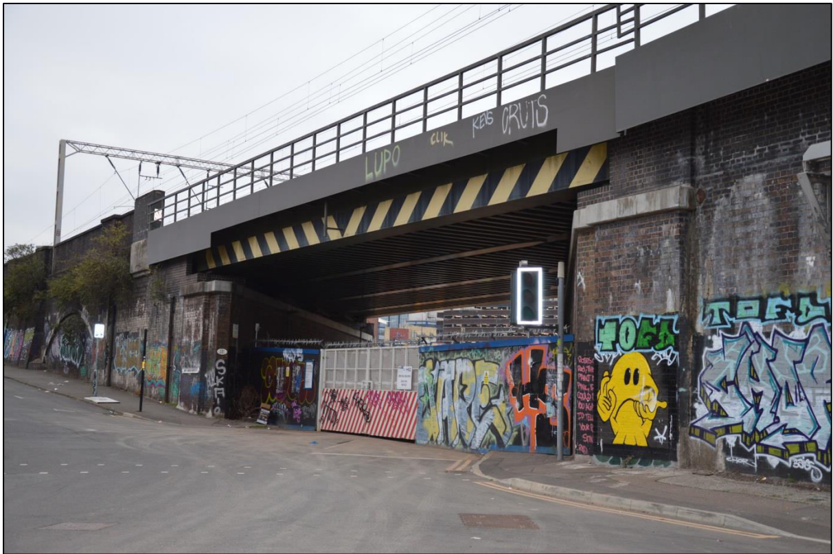
Fazeley Street Bridge (1986) as seen October 2025
