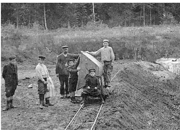
Above: A French light railway showing how it was just laid on the ground. Poor weather quickly caused it to subside and break up
