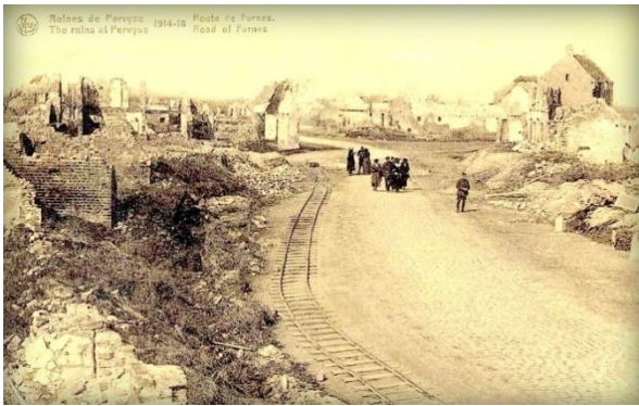
Above: A light railway at Pervyse, midway between Ypres and the Belgian coast. Note it is simply laid on the ground. the distortion is evident.
