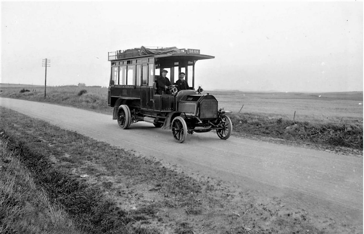
Above: SA614, a 1910 vintage Milnes Daimler operated by the Great North of Scotland Railway company, who also built the bodywork. It remained in service until 1924. The vehicle is seen in East Aberdeenshire near Newburgh where the company was providing a road motor service to Aberdeen in lieu of the originally intended branch line. The substantial bodywork was designed for the carriage of luggage and light goods on the roof and could seat a total of 18 1st and 3rd class ticket holders (Tom Ritchie Collection).
