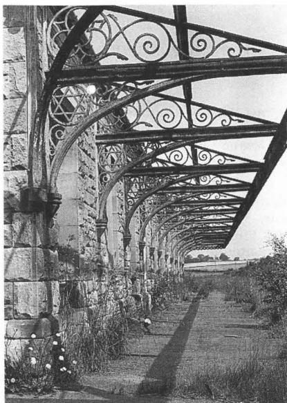
Whittingham station, NER: Alnwick-bound platform, shewing the decorative ironwork (Tim Edmonds)
