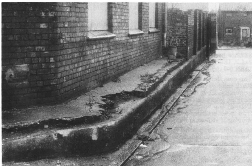
Figure 3. The only remains of the Ancoats branches. Large masonry blocks delineate the wharf at the end of the lower branch.
