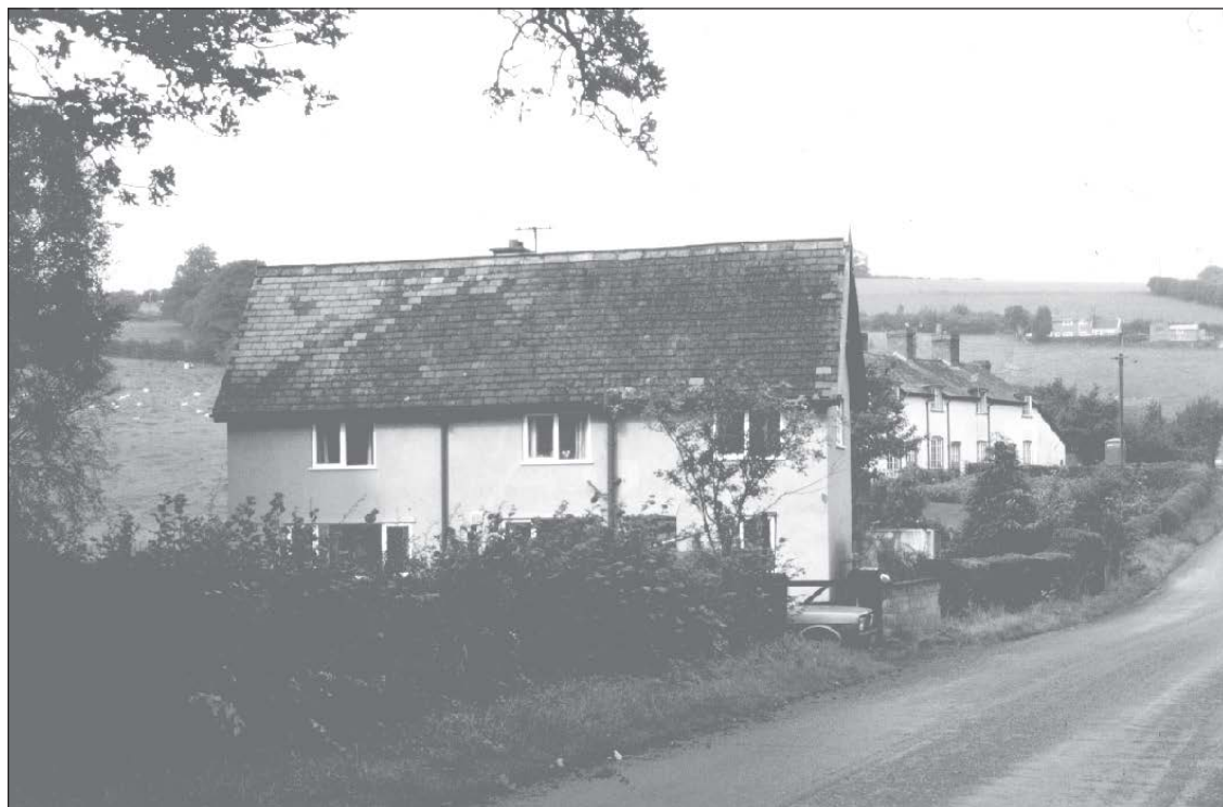
Cerist station building, 1982 (photographed by Tim Edmonds)
