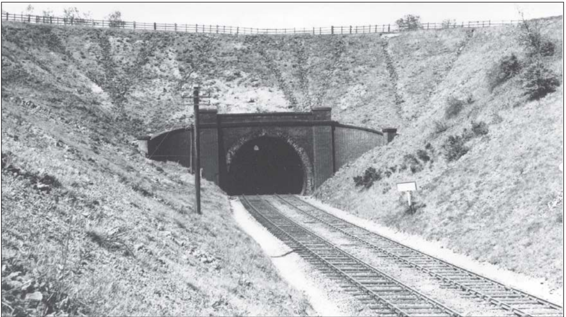
Below: South end of Hose Tunnel (834 yards), 4 June 1963
