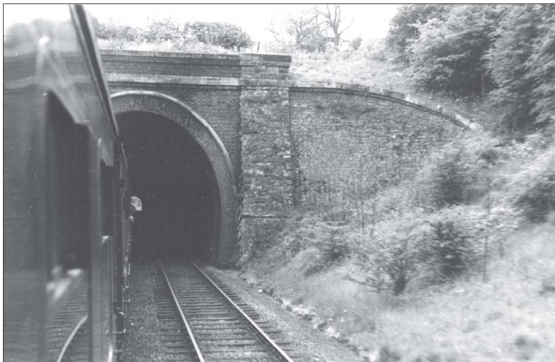
Entering the north end of East Norton Tunnel, 18 May 1863
