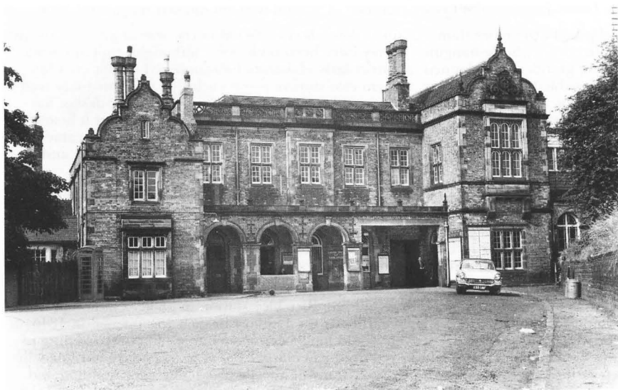
The frontage of Tamworth station, Trent Valley Rly by J. Livock, July 1958. Note mutilation of the colonnade
