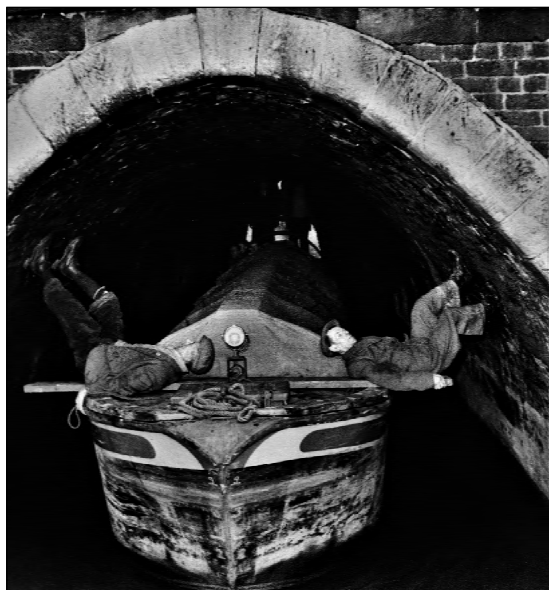
Figure 5. Boatmen Daniel Jinks (1899–1979) and Ernest Wood (1903–1986) demonstrate legging through Barnton tunnel on 28 February 1961. This is how boats were moved prior to the arrival of the steam tugs. The narrowboat being used for the demonstration is ‘Admiral’ class Lindsay which was built by W J Yarwood & Sons Ltd of Northwich for the British Transport Commission and launched on 4 May 1960 (yard no 922). It is still afloat and can usually be seen at the Etruria Industrial Museum, Stoke-on-Trent, having been donated by the British Waterways Board. [National Waterways Museum]
