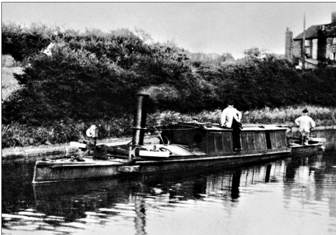
Figure 9. A steam tug at the north end of Preston Brook tunnel. Note the horizontal guide wheels extended to the front and stern of the tug which made contact with the tunnel walls.
