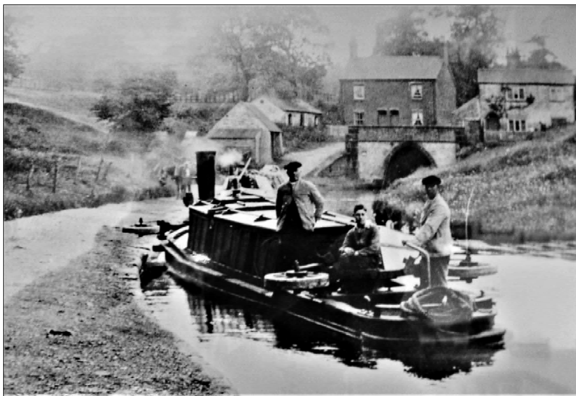
Figure 10. A steam tug at the south end of Preston Brook tunnel giving a clearer view of the extended guide wheels. [David Kitching collection]
