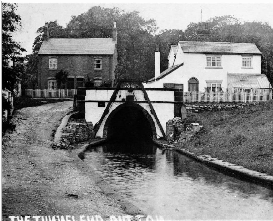
Figure 1. This is a close up view of the southern portal of Preston Brook tunnel. The houses were provided for the canal agent and two clerks. The bricks stacked either side of the tunnel mouth were presumably for repairs to the tunnel lining. [David Kitching collection]
