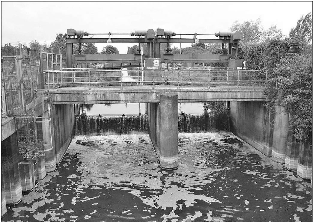
Bargate Sluice. From Google Earth, photo: Husssydogg (2009))
