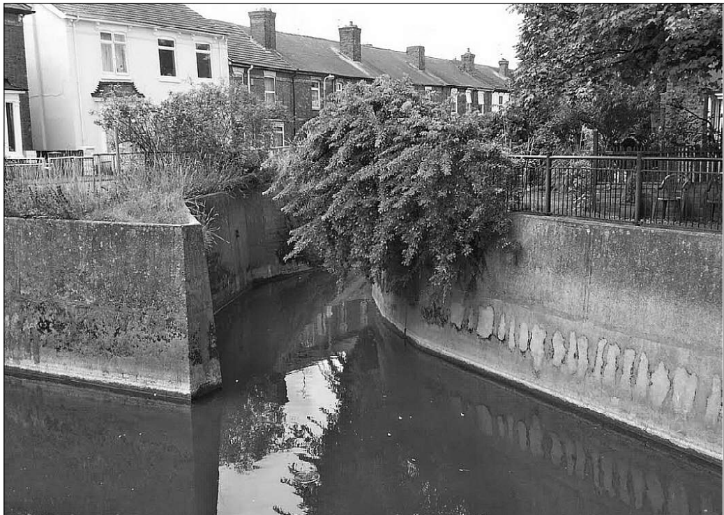
Great Gowts Drain outfall into Sincil Dike. (From Google Earth, photo: redimp 99 (2009))
