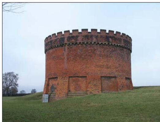
Fig. 49. A view of one of the two giant stacks for the ventilating shafts
