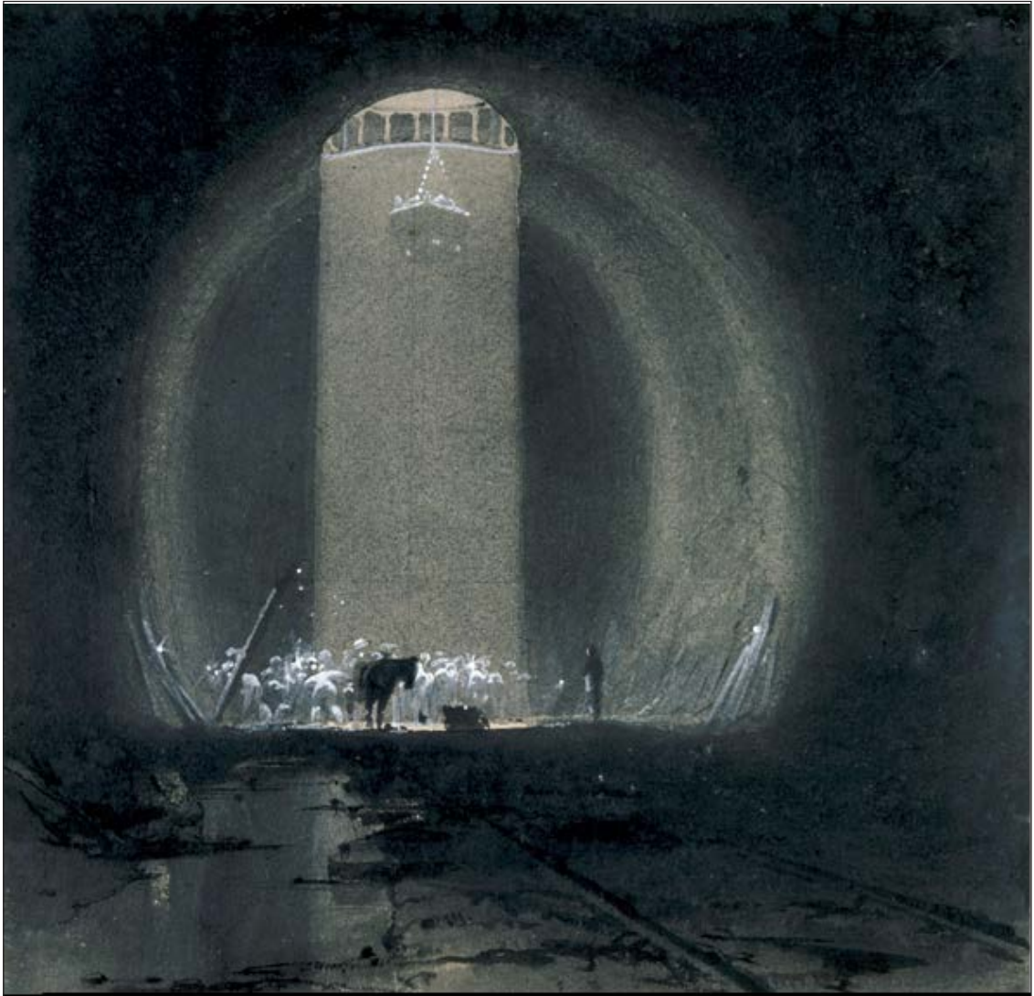
48a. Working shaft, Kilsby Tunnel, Northamptonshire, 8 July 1837 – wash drawing. National Railway Museum / Science and Society Picture Library (1990-7238)
