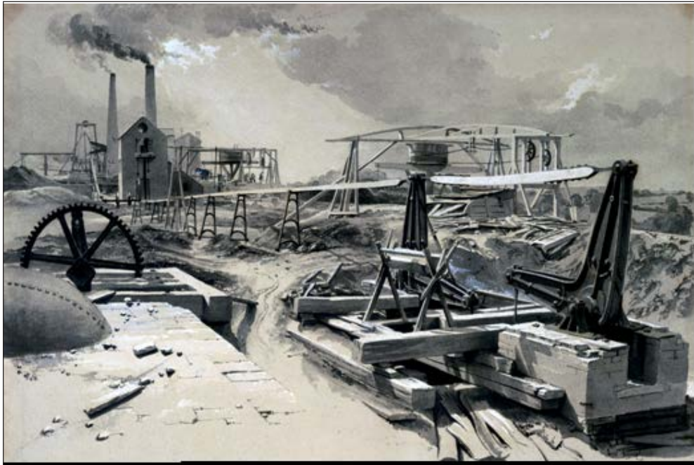
Fig. 50a Pumps, Ventilating Shaft, Kilsby Tunnel, Northamptonshire, 15 July 1837 – wash drawing. National Railway Museum / Science and Society Picture Library (1990-7241)
