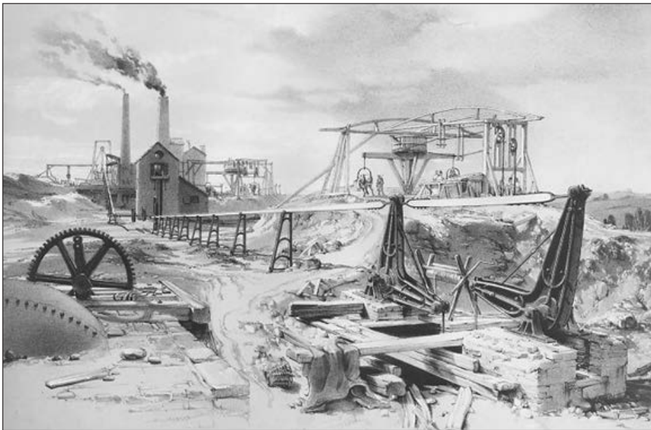
Fig. 50b Pumps for draining the Kilsby Tunnel. London, Published by the Proprietor J.C. Bourne, 19, Lamb's Conduit St and Ackermann and Co, Strand. Printed by C. Hullmandel. 1838
