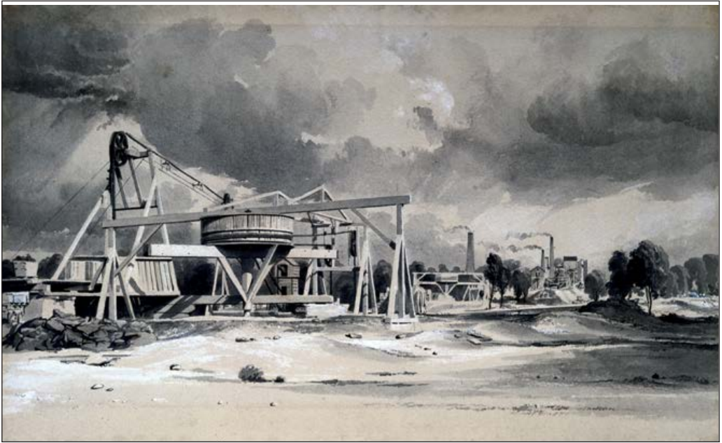
Fig. 53. Headgear and pumps at Kilsby Tunnel, Northamptonshire, 16 July 1837 – wash drawing. National Railway Museum / Science and Society Picture Library (1990-7242)
