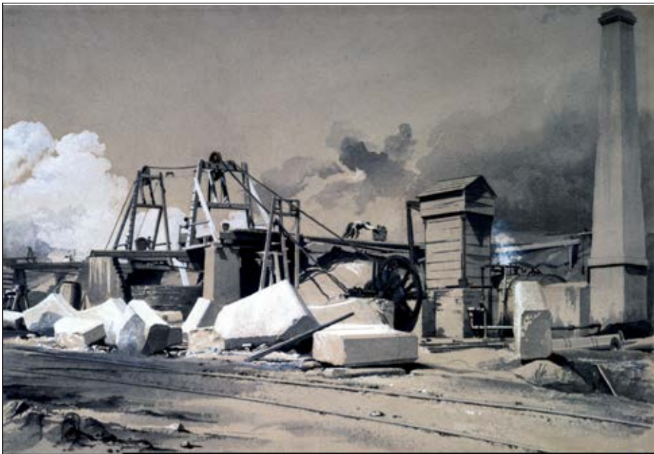
Fig. 52a. Ventilating shaft and winding engine, Kilsby Tunnel, 18 July 1837 – wash drawing. National Railway Museum / Science and Society Picture Library (1990-7243)
