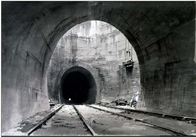
Fig. 47a. Great Ventilating Shaft, Kilsby Tunnel, October 1838 – wash drawing. National Railway Museum / Science and Society Picture Library (1990-7240)
