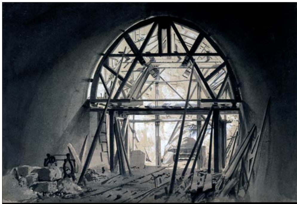
Fig. 46. North Church Tunnel, London & Birmingham Railway, 17 June 1837 – wash drawing. National Railway Museum / Science and Society Picture Library (1990-7219)
