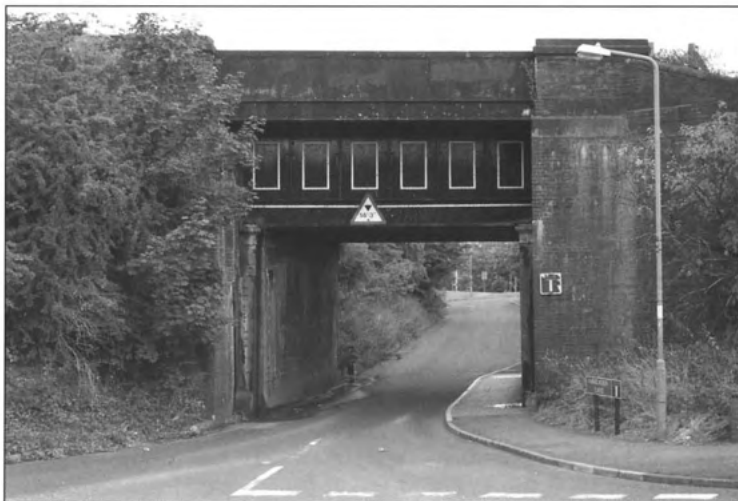
Iron aqueduct, Tame Bridge. This was the last aqueduct to be started on the Tame Valley Canal by the contractors Tredwell & Jackson. It crossed the parish road from West Bromwich to Walsall
