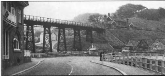
Figure 3: Sandsend Viaduct (J S Gilks)
