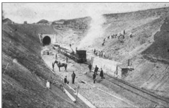
Figure 18: construction in progress at the south end of Grinkle [Easington] Tunnel (Whitby Lit. & Phil.)
