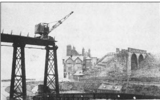
Figure 13: demolition of Sandsend Viaduct (K Hoole)
