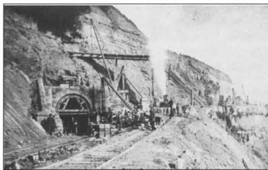
Figure 19: construction in progress at the south end of Kettleness Tunnel (Whitby Lit. & Phil.)
