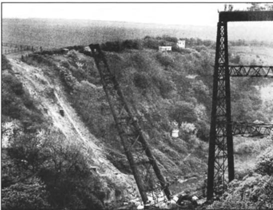
Figure 12: demolition of Staithes Viaduct [2] (British Rail)
