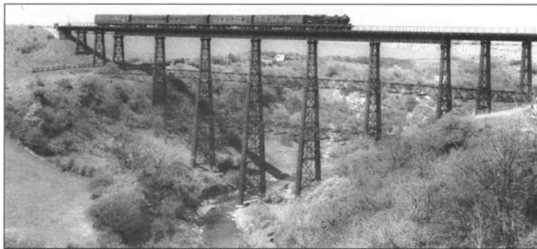
Figure 4: Staithes Viaduct (N E Stead)
