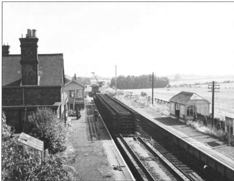
After closure of the line between Bedford and Cambridge on 1 January 1968 there was little delay before most of the track was lifted. This was the scene at Old North Road Station on 22 August 1968, with demolition proceeding towards Cambridge
