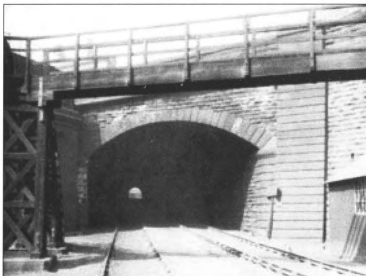
Spital Hill Tunnel lower portal from Wicker Goods Yard, looking north west. Photograph by Sheffield City Highways Department, Bridges Section, July 1929 (Sheffield City Council Archives and Local Studies Service) Examination of the original image shows that the original ascending line (to the left) was almost certainly out of use by this time. At the top end there is a wagon on the track, almost certainly a cattle truck, as this section was by then used by the GC/LNE as a siding serving cattle pens. Bridgehouses goods depot can be seen beyond that.
