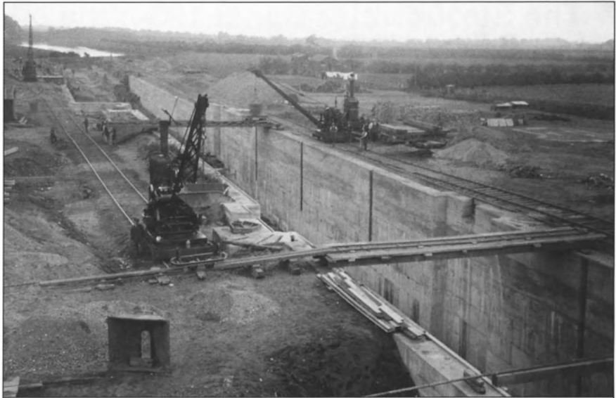
In making the concrete walling steam cranes working along the sides moved materials and excavation spoil. There were also some hand-propelled waggons on c.2 ft track
