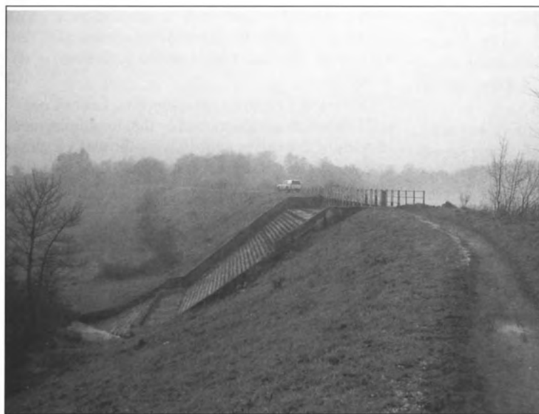
Auxiliary spillway built in 1935 over the headbank of Townhead Reservoir, Kilsyth
