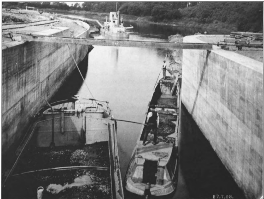
Narrow boat, barge and dredger at the lock as the link channels are dredged out
