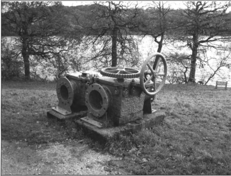
The preserved box valves at Knypersley Reservoir
