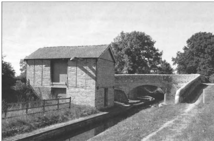
The Ellesmere Canal at Rednal, a length of canal cut by James Houghton
