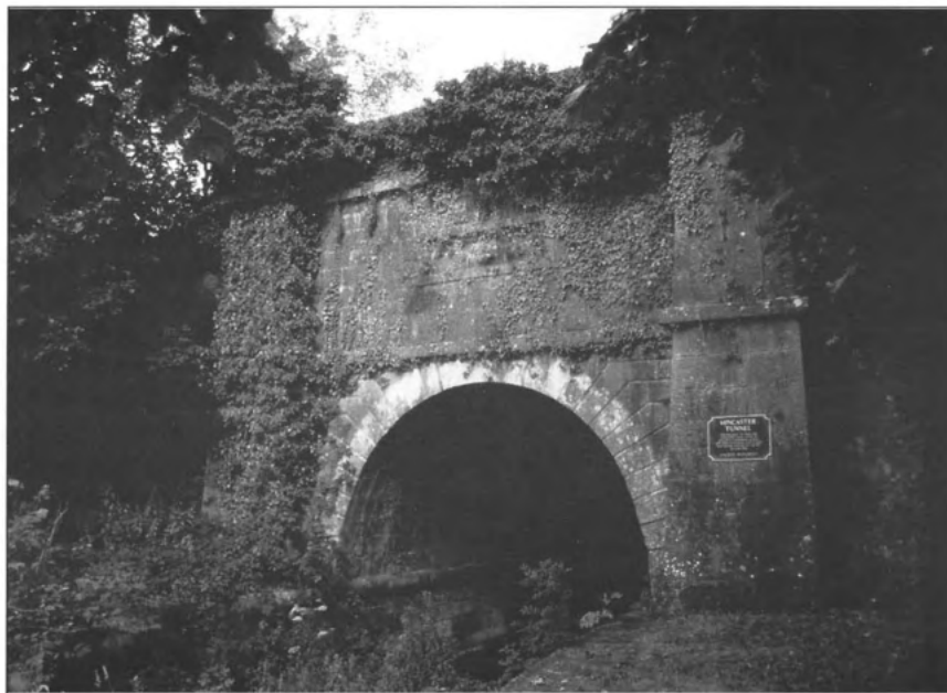
Hincaster Tunnel, one of those built by Daniel Pritchard
