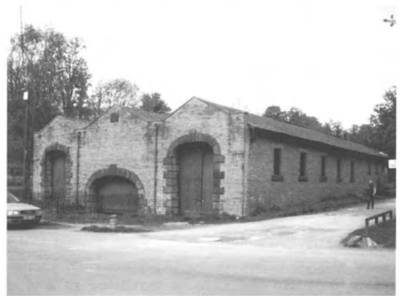
The differences in the windows show the two construction phases of the Whaley Bridge warehouse. The nearer, original end was later allocated exclusively to German Wheatcroft after the farther end was built for use by Pickford & Co.
