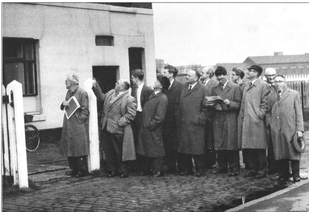
An RGHS North West Group party in 1962 at 'The Three Pigeons', Dallam, Warrington, reputed to have provided a booking office and waiting room for the Warrington & Newton Railway
