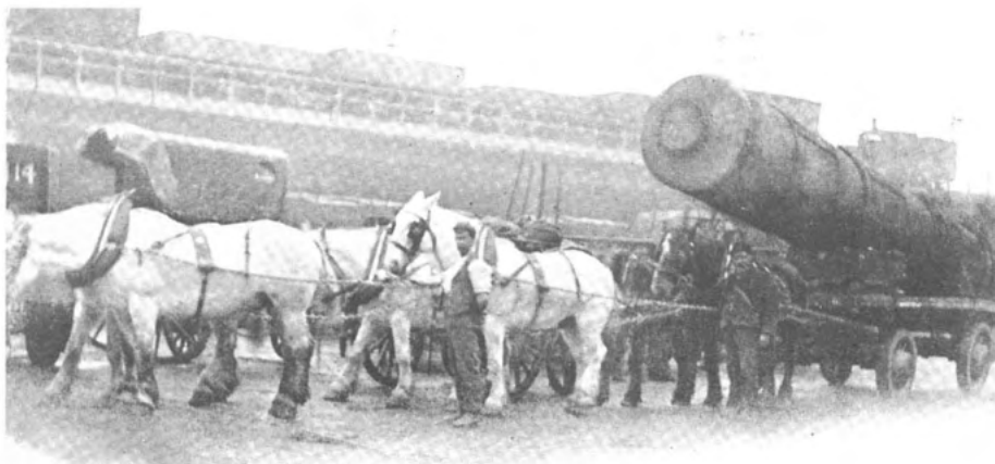
Carting a big boiler, L&NWR
