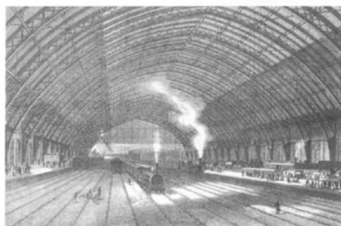
St Pancras Station roof
