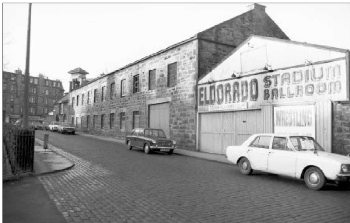
Figure 4. Leith Engine Works, nos 1-3 Mill Lane, showing the Mill Lane frontage of the works from the south-east. The two-storeyed building probably housed the light machine shops. [© HES. Reproduced courtesy of J R Hume. SC 784513]
