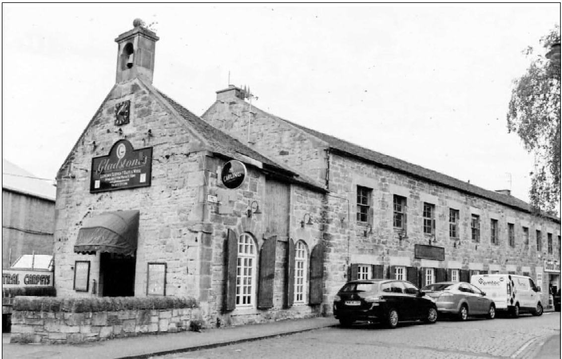
Figure 3. The surviving part of Leith Engine Works in Mill Lane. [Robert Humm, 19 May 2017]
