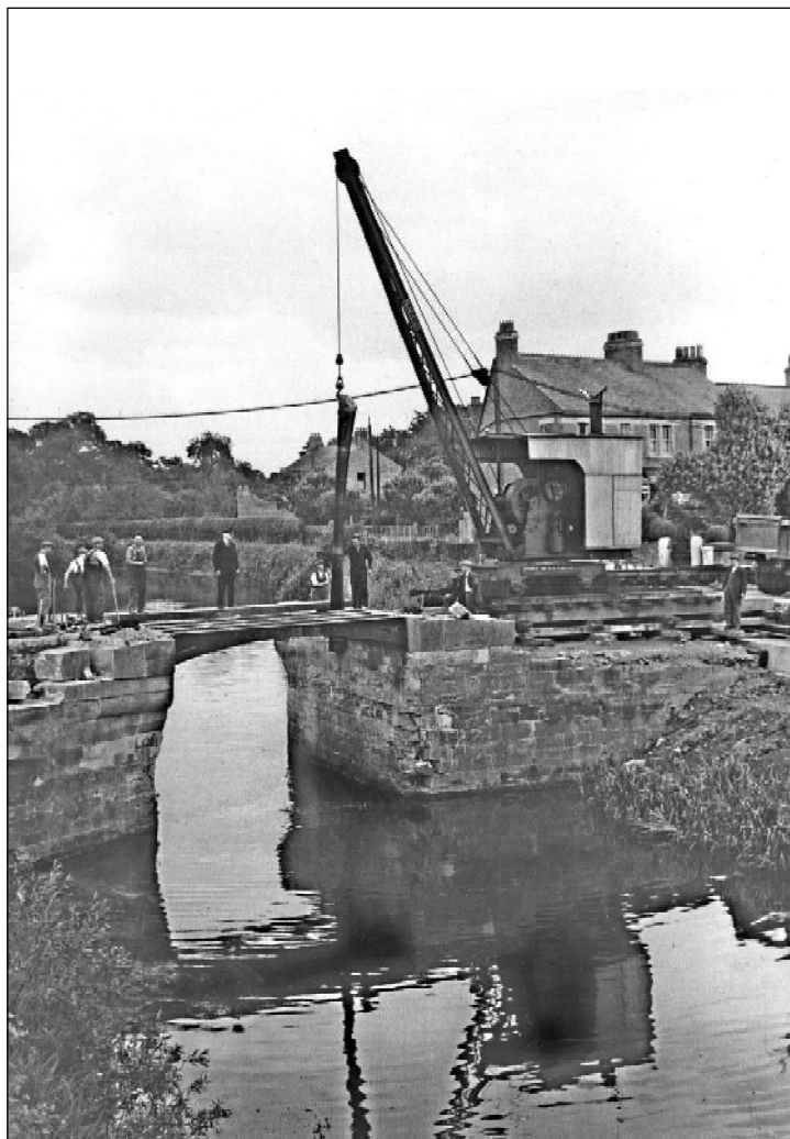
Figure 5. The old bridge stood where the downstream bridge forming part of the roundabout now stands. A news item from The Engineer of 2 August 1946 implied it was being dismantled in July of that year; therefore the temporary bridge that later formed the upstream part of the roundabout must have been in operation by that time. [Photograph by 'Chief Civil Engineer [BR] NER York']
