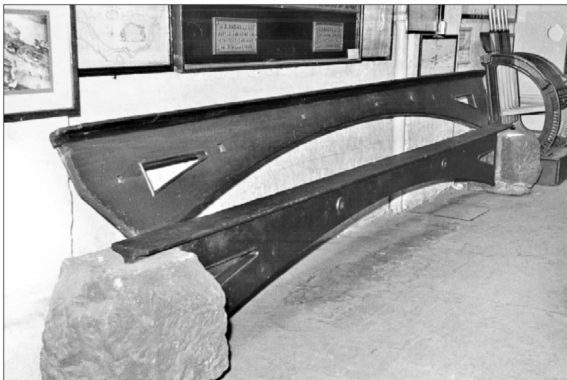
Figure 6. Two of the cast-iron girders on display at the then LNER's Queen Street museum. Note that the bearing stones had been reduced in size, and that the girders were not cast from the same pattern. The ringed holes for tie rods had been omitted from the pattern from which the upper girder was cast. [Photograph courtesy of James Carter, the Science Museum's Freedom of Information Officer]
