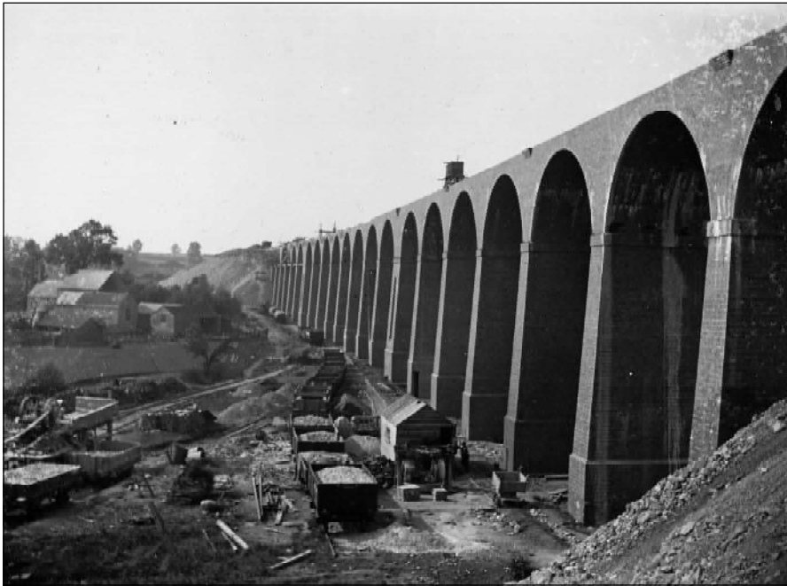
Figure 6. Brackley viaduct in July 1896. Details shown in the contractor's yard below include a stone crusher and clay pans.
