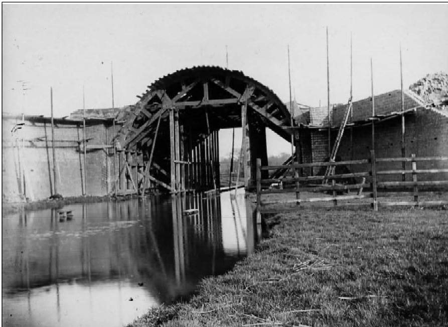
Figure 7. A massive arch of timber centring stands ready to support the brickwork of the bridge over the River Swift at Lutterworth.
