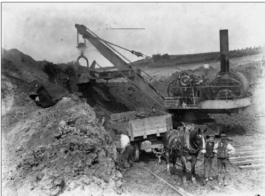
Figure 8. On the GW&GC Joint line between Wotton Underwood and Haddenham, Newton took several photos of this excavator and the young lad with his horse and tipping wagon. By now (c1903) he was using a half-plate camera, giving a much more detailed image.
