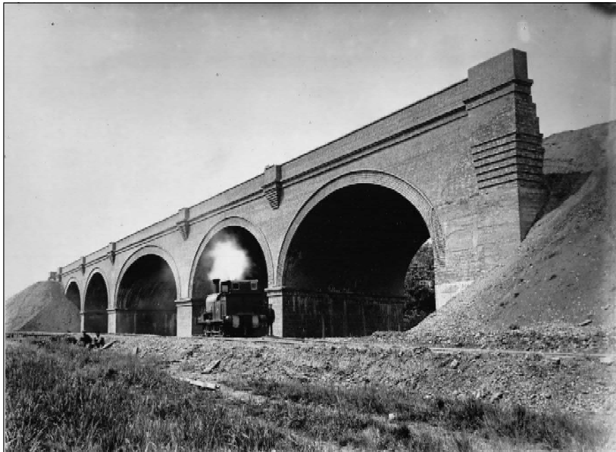
Figure 9. The freshly completed brickwork of Denham viaduct, c1903. The locomotive is Cefn (Hunslet Engine Co, no 256, 1881) of contractors Pauling & Co.
