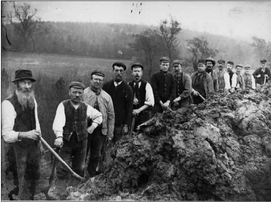
Figure 4. One of the photographs Newton planned to use in his article on the London extension. It shows workmen on the embankment between Rothley and Quorn, on a section of the line now preserved by the present Great Central Railway.
