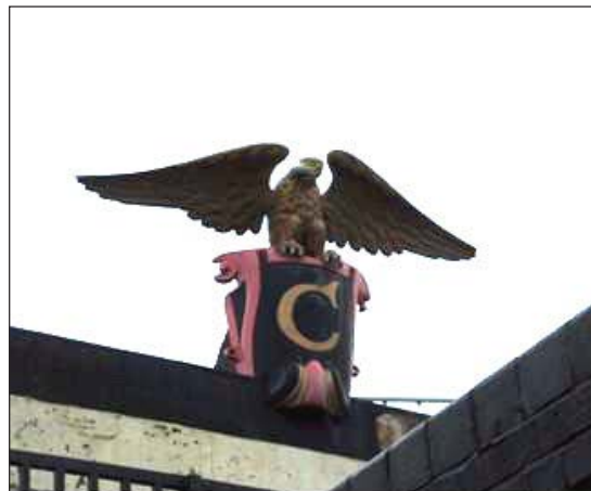
Fig. 1. An eagle atop the 1940 'bomb-proof' Crewe North signal box, inside Crewe Heritage Centre
