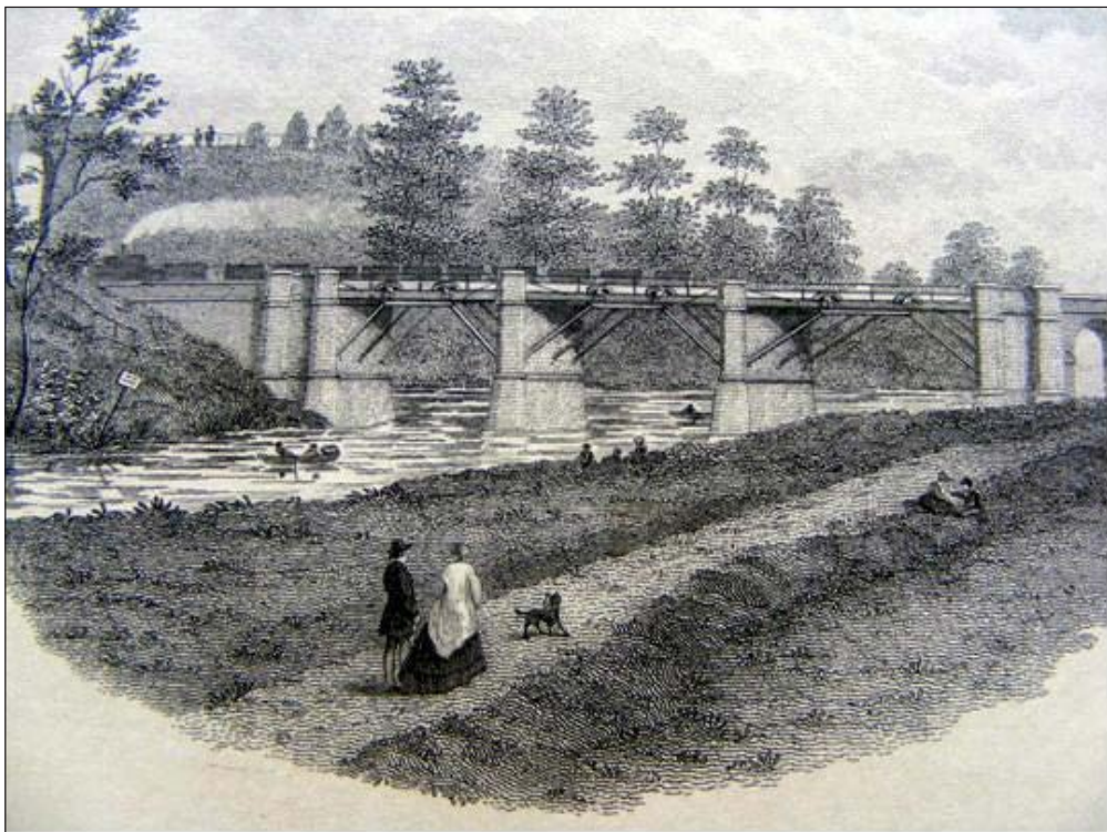
Fig. 8. Engraving of 1853 by John Romney showing the rebuilt Dee bridge. Note that the eagles have been reinstated.
