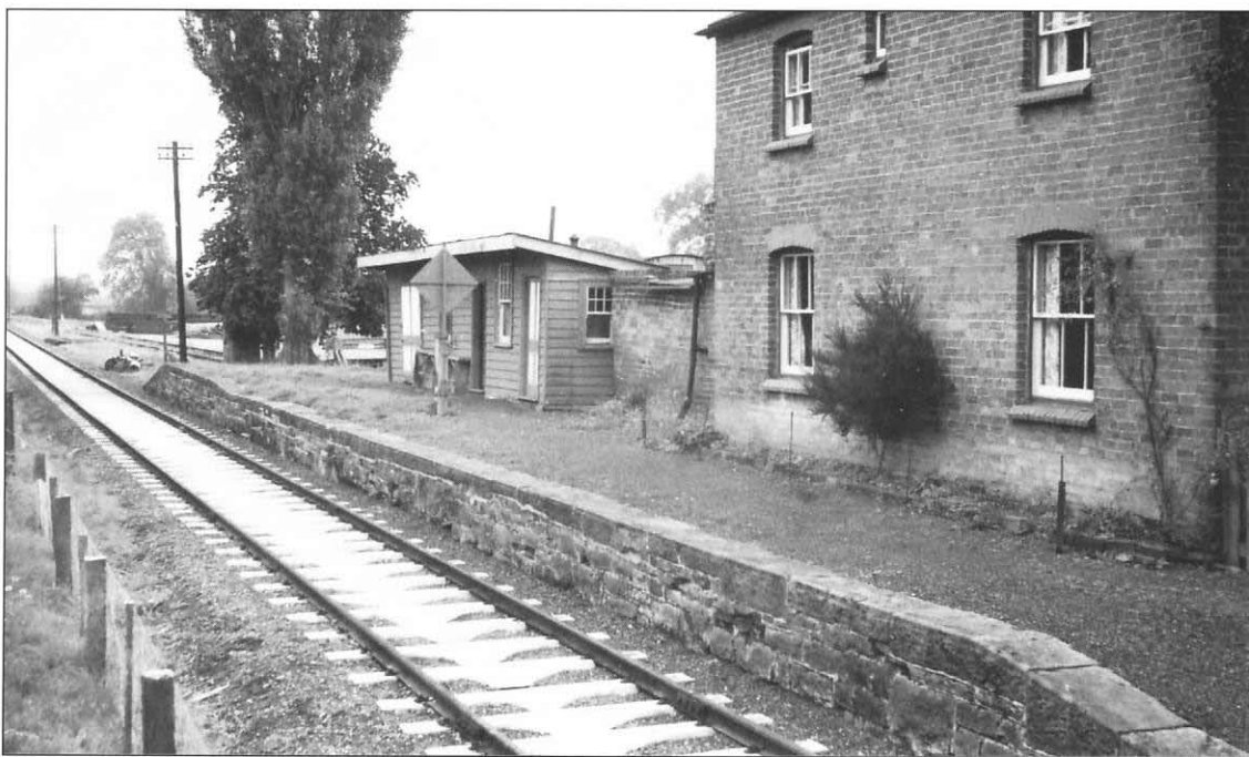
Maesbrook Station survived in its PS&NWR form into the modern age. The station house, building and platform are probably from the former period. The stop sign was added in the Stephens' era; the track was laid by the military after 1941.
