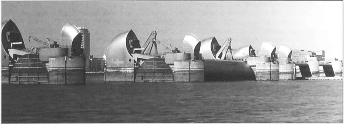
The Thames Barrier viewed from downstream. The large rising sector gate in the centre is raised to its 'operating' position, whilst the gate to the left of it is in its 'rest' position, close to the river bed. (Photo: Henry Gunston, September 2004)
