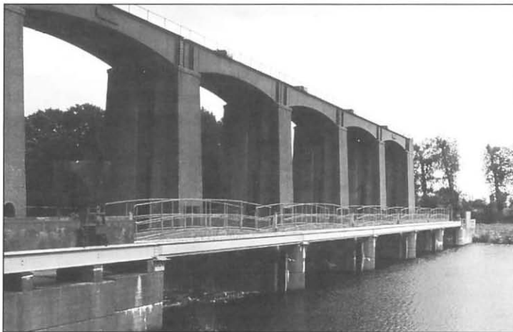
Holme Sluices on the river Trent below Nottingham, from upstream. The plate on the nearest span carries the name 'Ransomes and Rapier'
