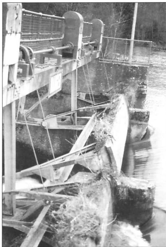
Three-bay radial gate structure on the Thames at Sutton Courtenay (near Culham). The far gate is closed and the centre gate lifted clear of the water. Note trash lodged during overtopping when flood flows have occurred.
