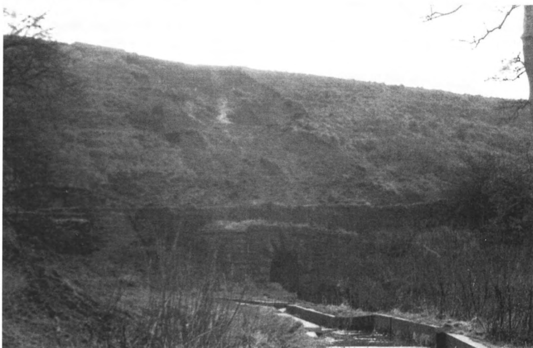
COOMBS BROOK RESERVOIR BREACH 1976
