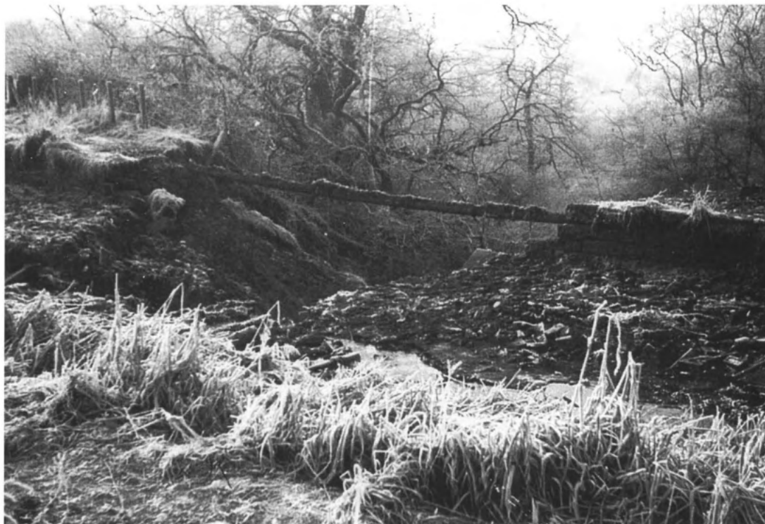
CAPTAIN CLARKES BRIDGE BREACH 1973
