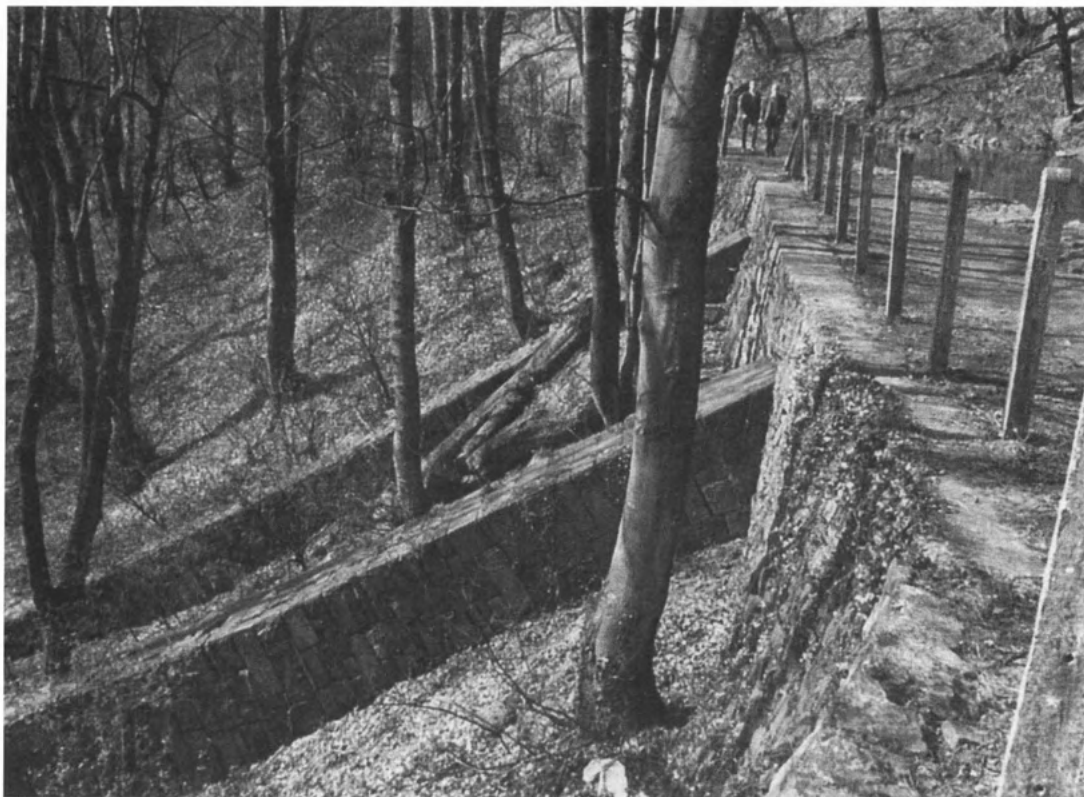
GASKELL WOOD CULVERT BREACH 1833
