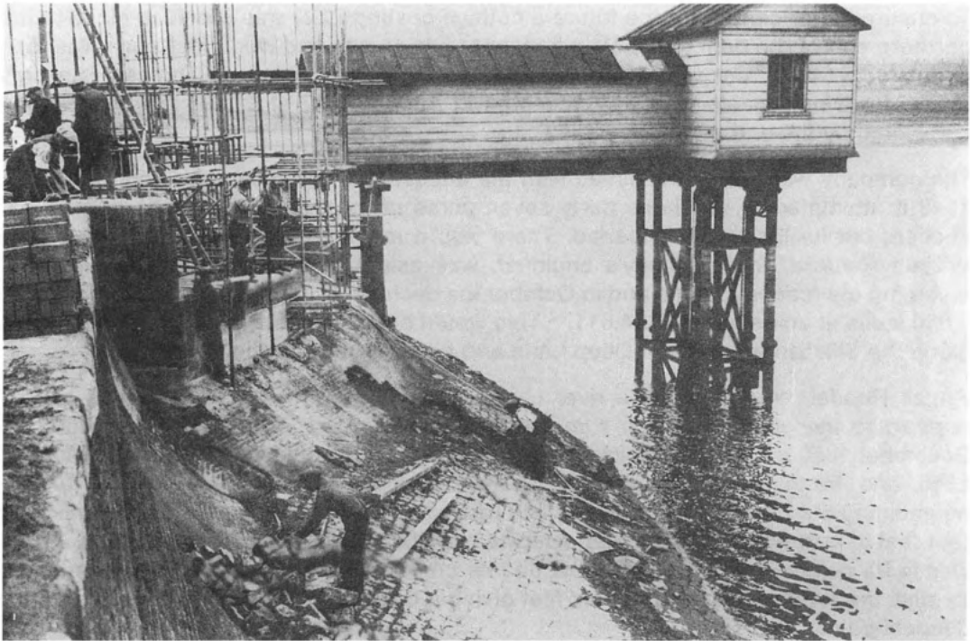
To enable the syphons to be installed the water level in the reservoir had to be lowered for a few weeks. The sluice house is little altered today. (Waterways Archive, Gloucester)
