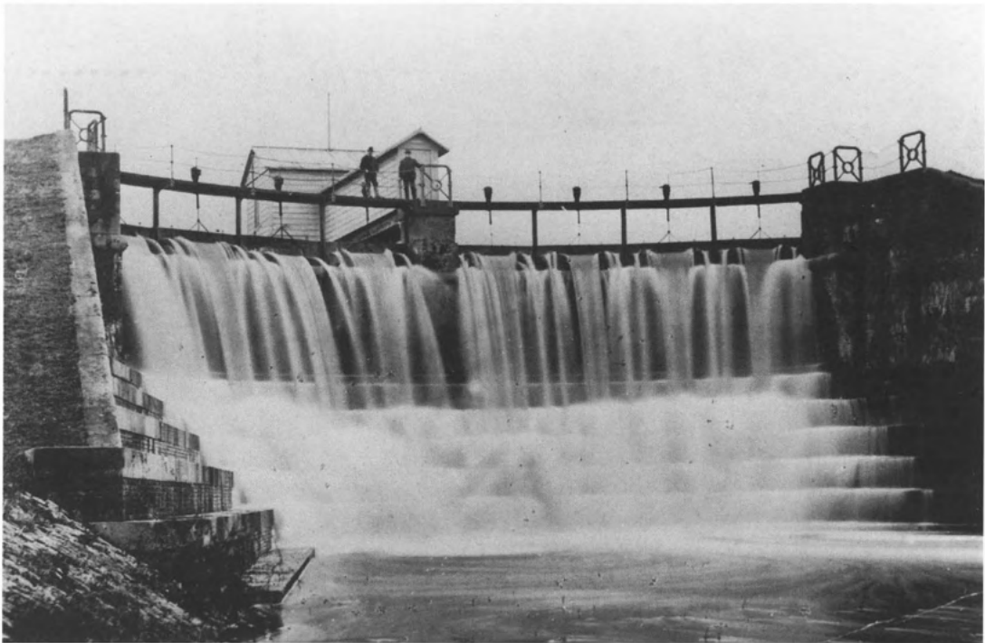
The Welsh Harp dam about 1890 showing water being released through the original sluices along the crest of the weir. (Brent Council, Cricklewood Archive & Library)
