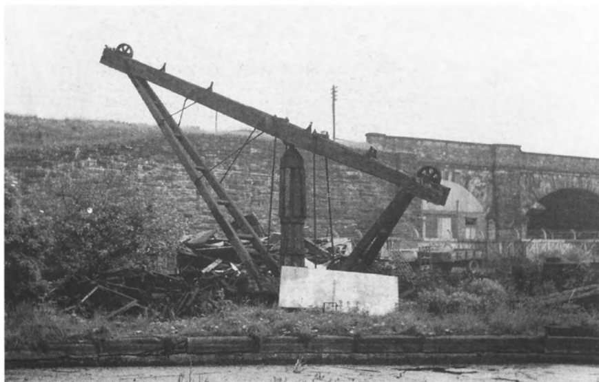
6 June 1965, looking east across the canal at the only (at this date) surviving cantilever gib crane in a nearly complete and operational state, but without its cargo chain. This crane carried three notices, one showed 'GCR C285' and was the Great Central Railway crane inventory number, with the other notices giving weight and use restrictions.
