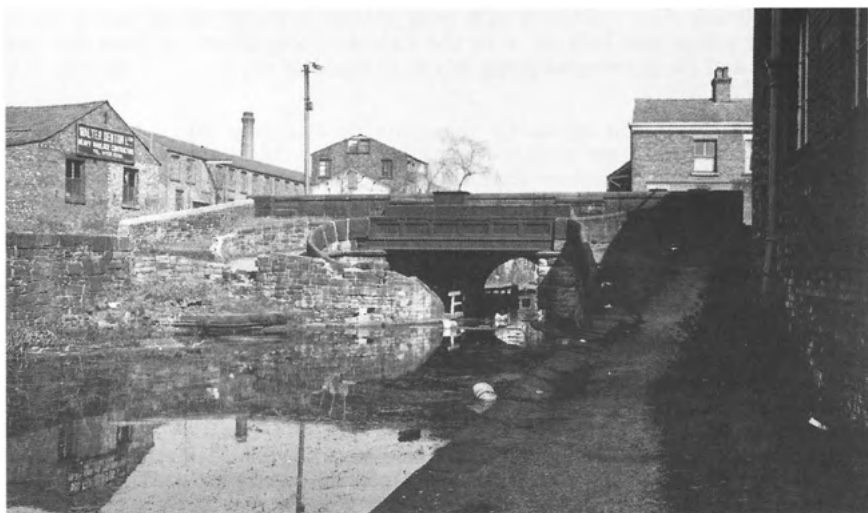
12 April 1968, looking north at Hyde Lane (now Manchester Road) change-bridge built after representation by the Trustees of the Hyde Turnpike in 1834. The building at the left was the former office of the Hyde Lane and later Hyde and Houghton, Colliery, 1795 to 1889.
