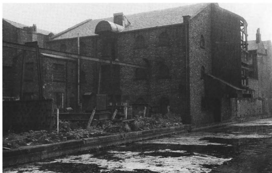
6 June 1965, looking south east across the canal towards the 1828 warehouse and showing the covered canal side loading way and the 'cat-head' on the north side of the warehouse. Note the small semi-circular windows that were a typical feature of canal and river warehouses at that date.
