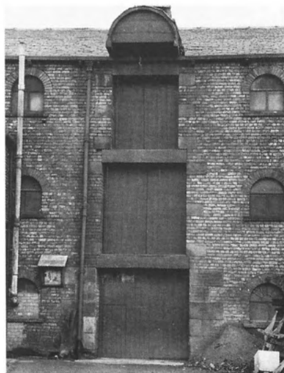
17 March 1968, looking south at the three-storey 1828 warehouse loading way access doors with the 'cat-head' still complete under the arched cover. The small notice board at the lower left carried an LNER warning notice. Note the small semi-circular windows.
