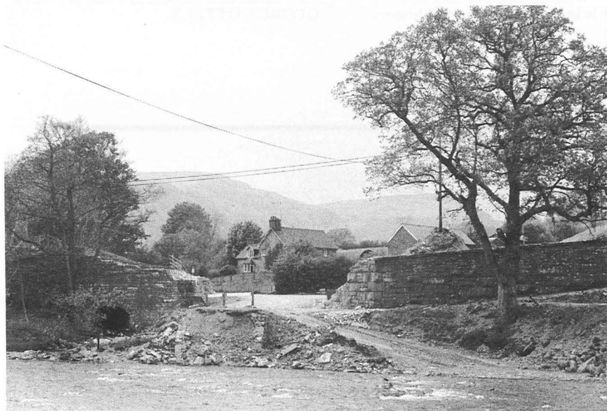
Remains of the Elan Valley Railway overbridge at Dolafallen near Rhyader, recently demolished in connection with rebuilding of the road bridge over the River Elan. (Tim Edmonds)
