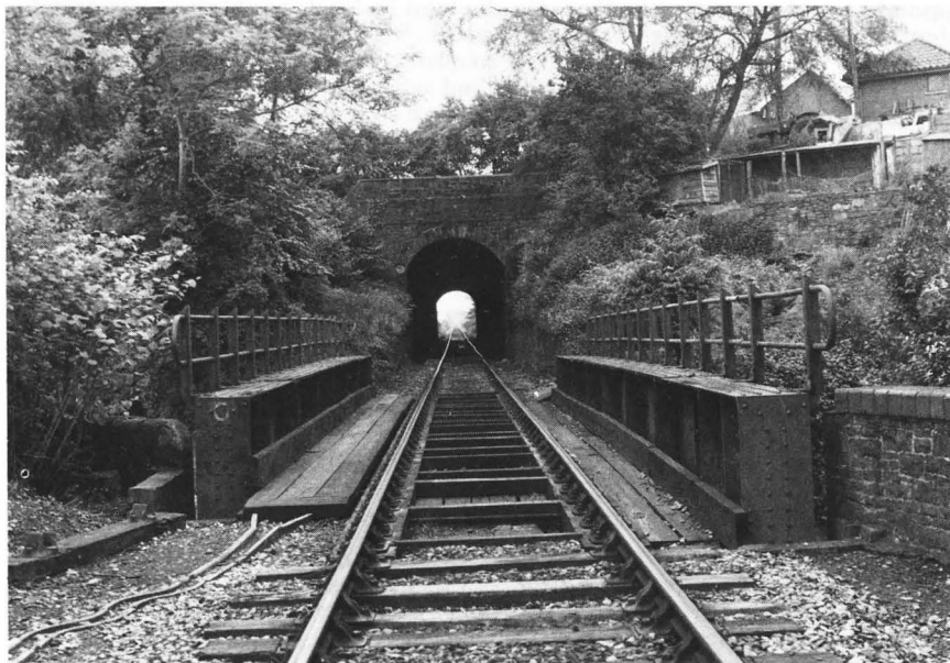
Pontarddulais Tunnel from north end, prior to installation of paved track, shewing the bridge over the River Loughor, into which water from the tunnel is drained
